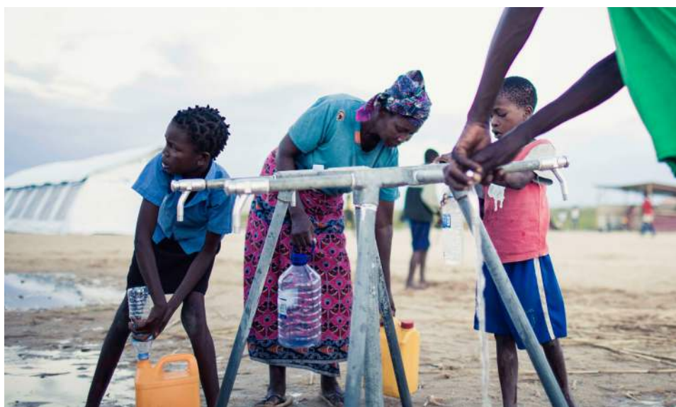
In the Beira IDP camp, a family has access to clean water through the system built by Oxfam. Credit: Micas Mondalane/Oxfam
